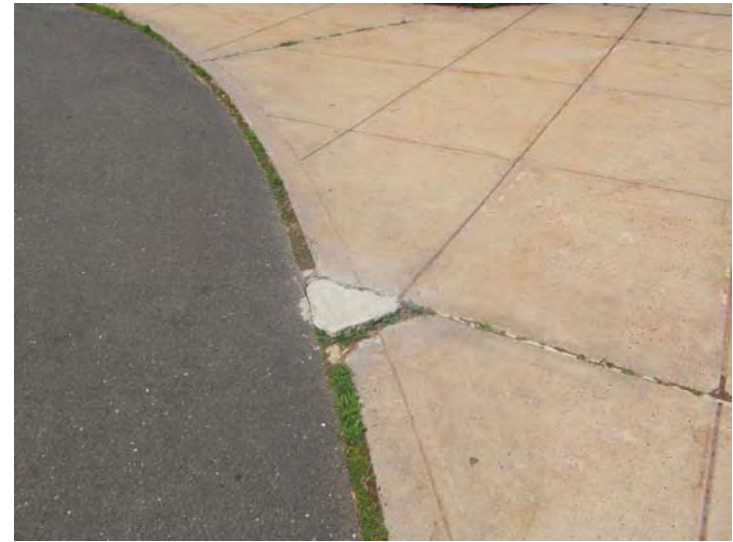
Isolated areas of cracking were noted within the concrete sidewalks present on the property.
