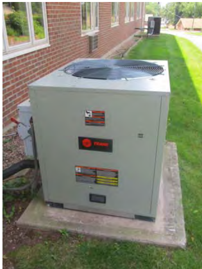
Newly installed air cooled condensing unit located at the east end of the building.
