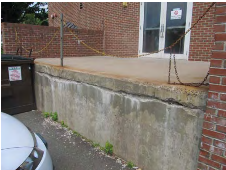
View of spalled concrete at loading dock area.
