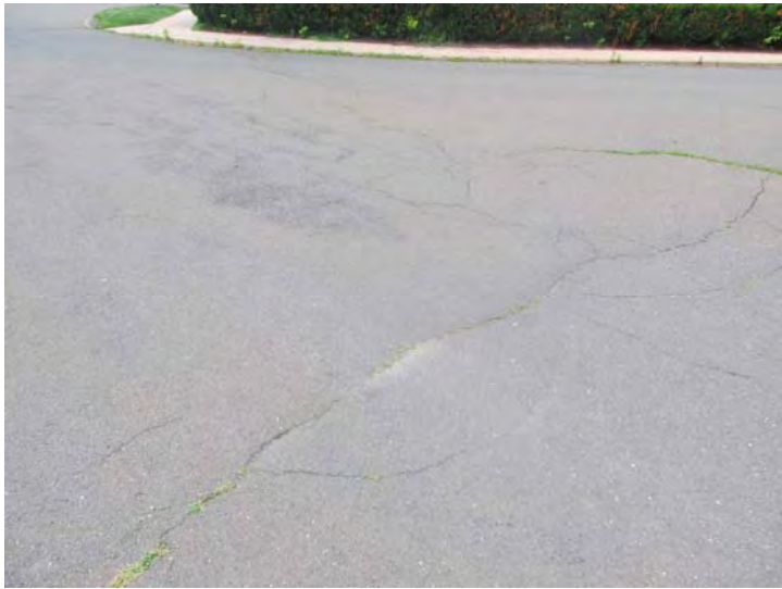
Localized areas of pattern cracking were noted within the asphalt paved surfaces, most notably at the entrance driveways and surface parking areas.
