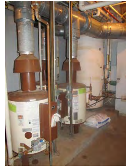
AO Smith 'Burkay' boilers and vertical storage tanks serve the building's domestic hot water needs.
