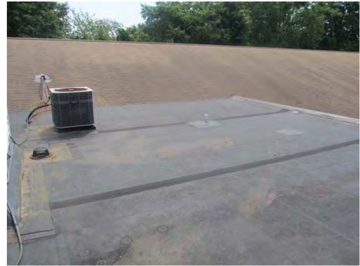
View of fully-adhered single ply roof membrane.
