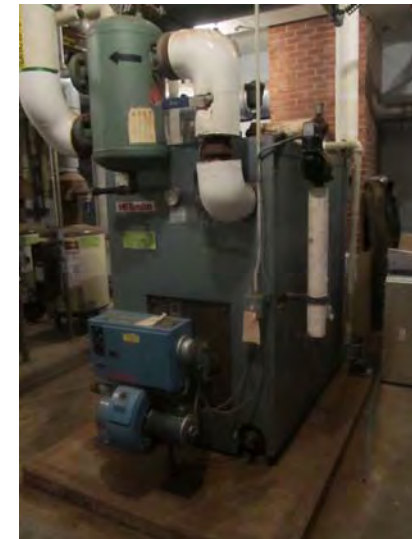
Natural gas fired HB Smith boiler for production of hydronic heat.
