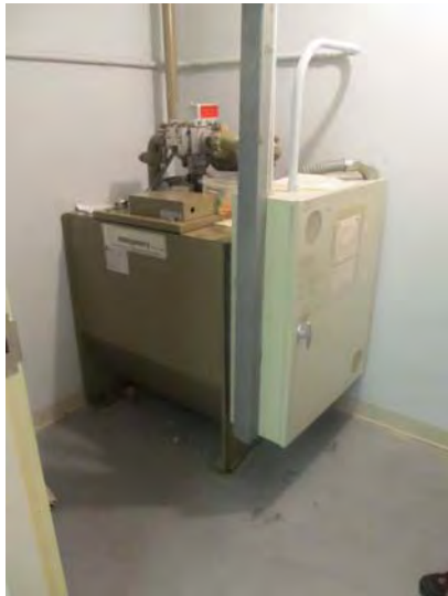
Hydro-mechanical pump and controller/dispatcher unit for elevator.
