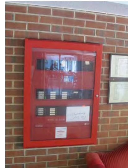
Original zone-type fire alarm control panel monitors and supervises common area end devices.
