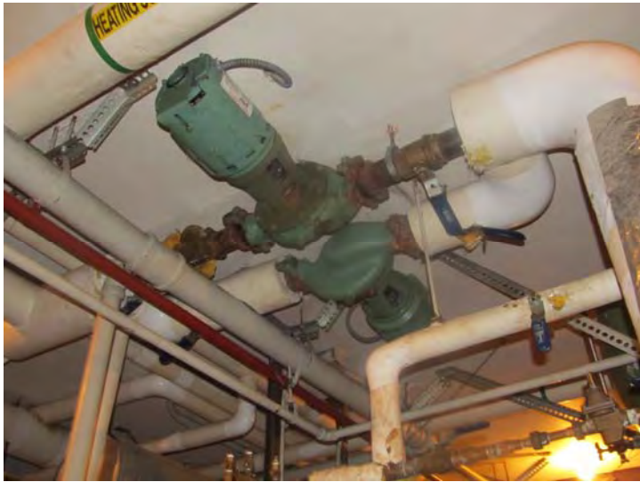
Inline circulation pumps for hydronic heat – Both to be replaced in 2013 per management.
