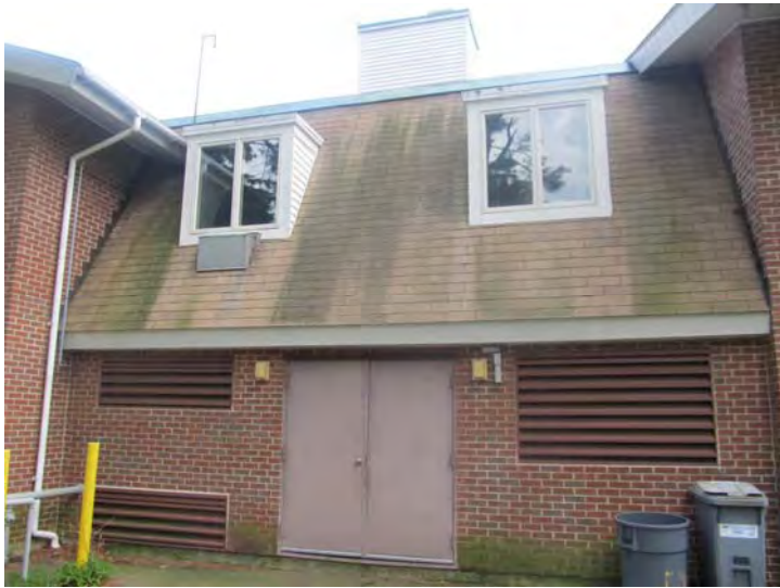
Pronounced staining noted on some asphalt shingled roof areas and isolated missing/deteriorated asphalt shingles also noted.
